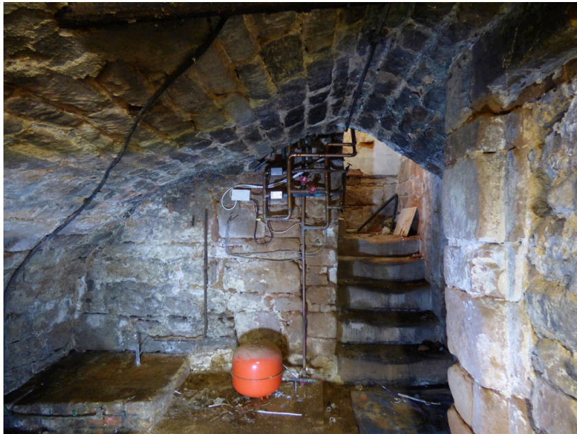
Fig. 6. Current entrance to the cellar, cut through the original S wall.
