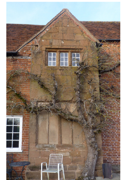
Illustration 10: Traceried window head at Cryfield Grange Photographed on 22/2/2017 by N. W. Alcock
