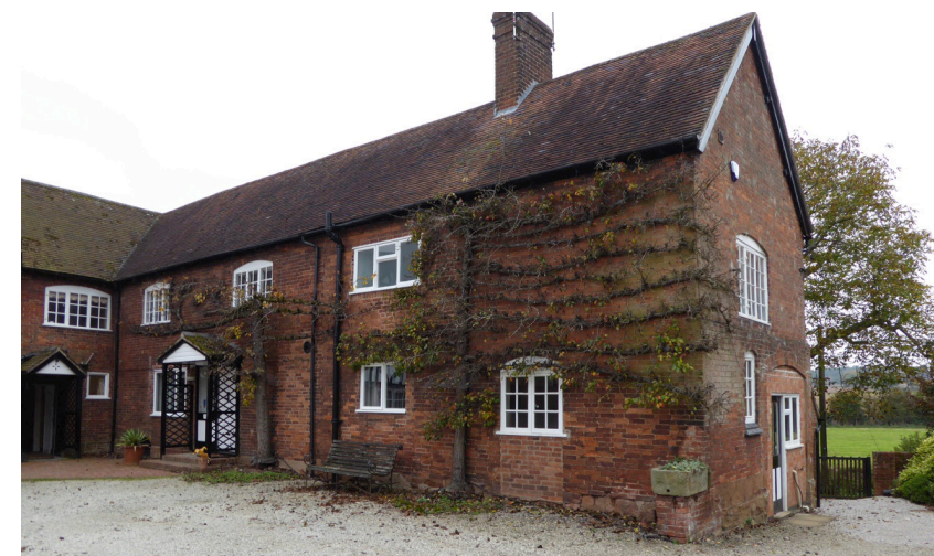
Fig. 1. The N range of Cryfield Grange, from the NE.
