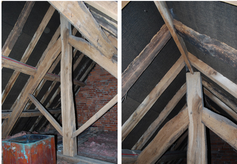
Fig. A3. The early nineteenth century roof structure in unit C (photos James Edgar) (a) Whole truss; (b) Apex of king post (smoke-blackened rafters in foreground)
