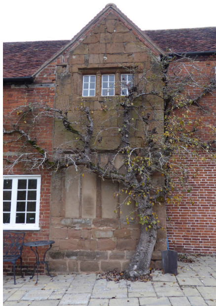
Fig. 10. The stone 'tower' on the S range.
