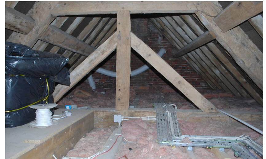
Fig. A5. Truss of unit B, probably early-mid eighteenth century (Photo James Edgar).
