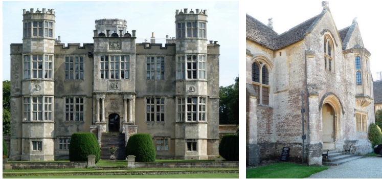
Fig. 9. Great Chalfield, right, and Barlborough Hall, showing their porches.
