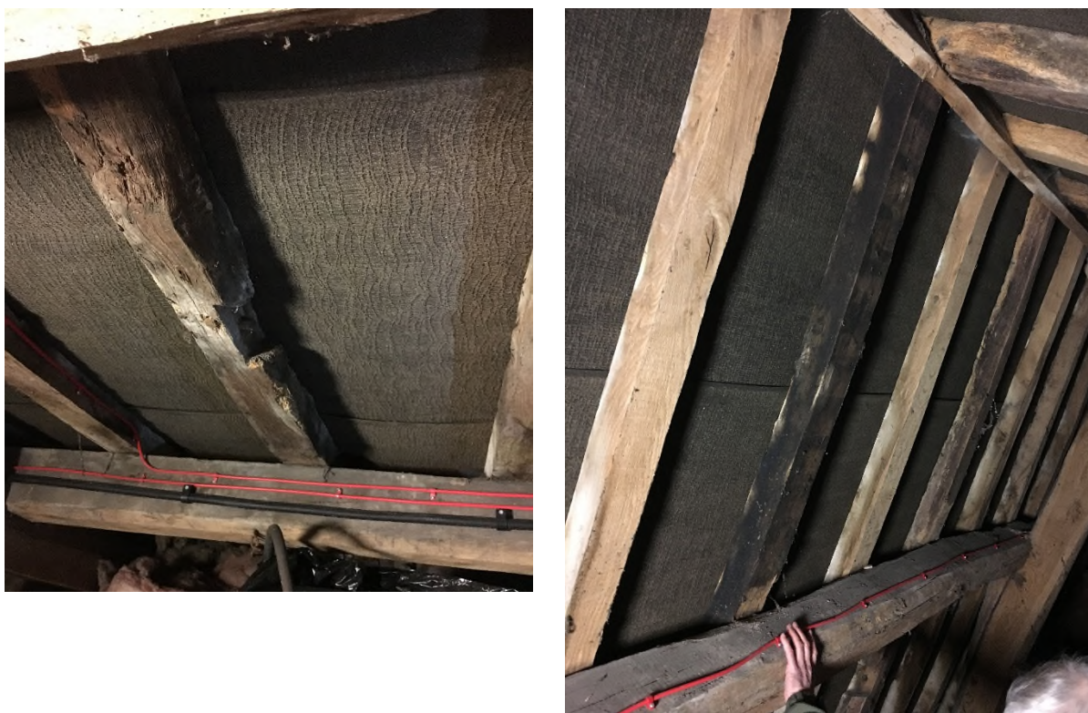
Fig. 5. (a) [left] halving in reused rafter; (b) [right] heavily smoke-blackened rafter. [Photos: Alex Russell]
