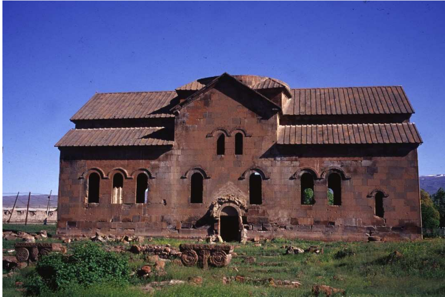
Fig. 2 Southern façade of Aruch (670) with capital from palace in foreground
