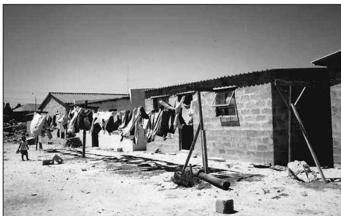
Capetown, South Africa. Homes self-built by a housing federation.
