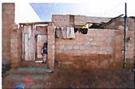
(a) Block masonry house in Karachi [8]
