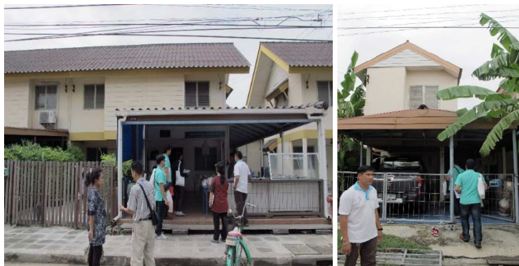
Figure 6.3 NHA houses which are between 5-10 years old
