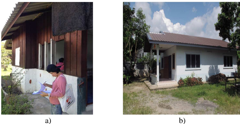
Figure 2. A one-storied house of concrete block and cement and wood and a) and a house of concrete block and cement (b).
