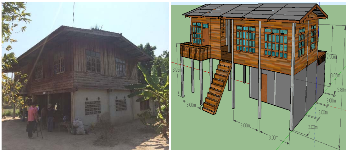
Figure 2.11 2-storey house constructed by concrete and wood of Central Thailand.
