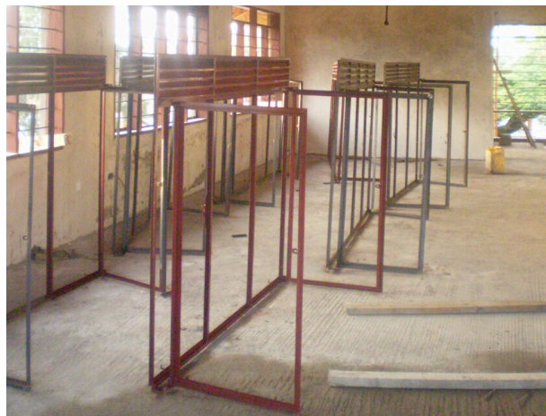
Figure 5: On site construction of steel window frames
