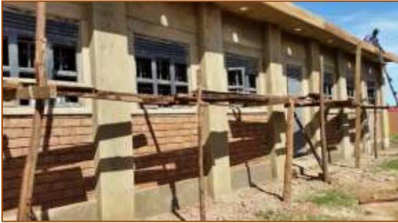
Fig. 11: ISSB house (60 % plaster)
