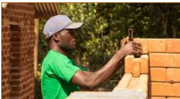
Fig. 9: Dry stacking to save mortar
