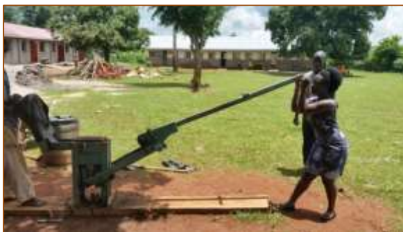
Fig. 7: Onsite ISSB production
