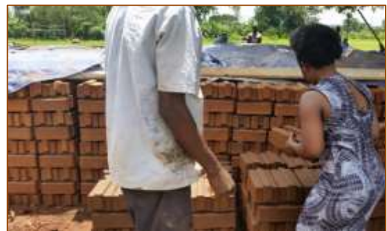
Fig. 8: Stacking and curing of the blocks
