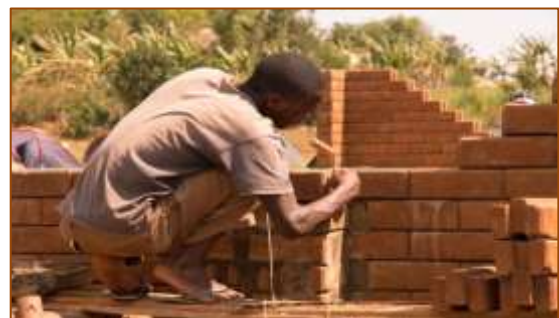
Fig. 10: Mortar applied in columns
