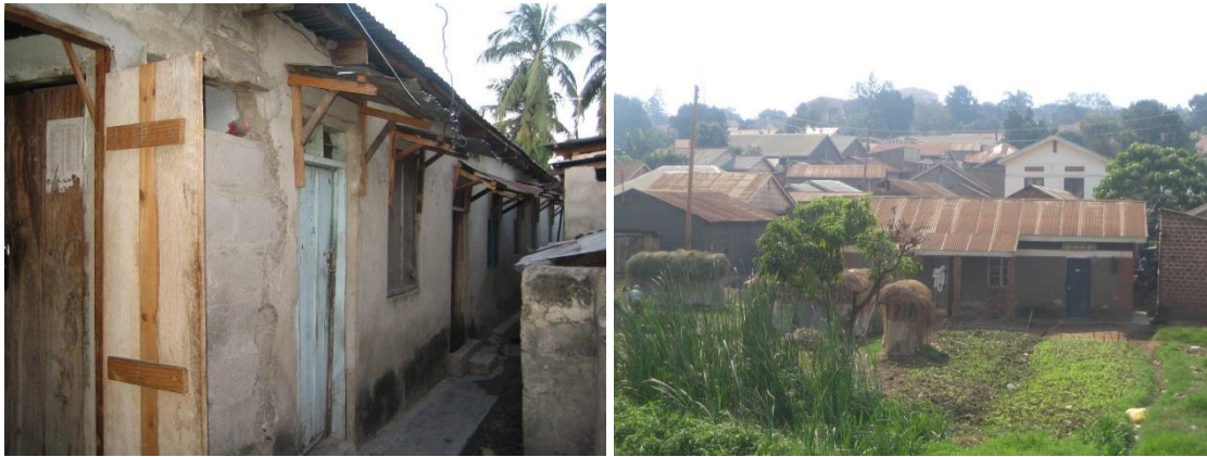
Figure 1: low-income housing with iron sheet roofing.
