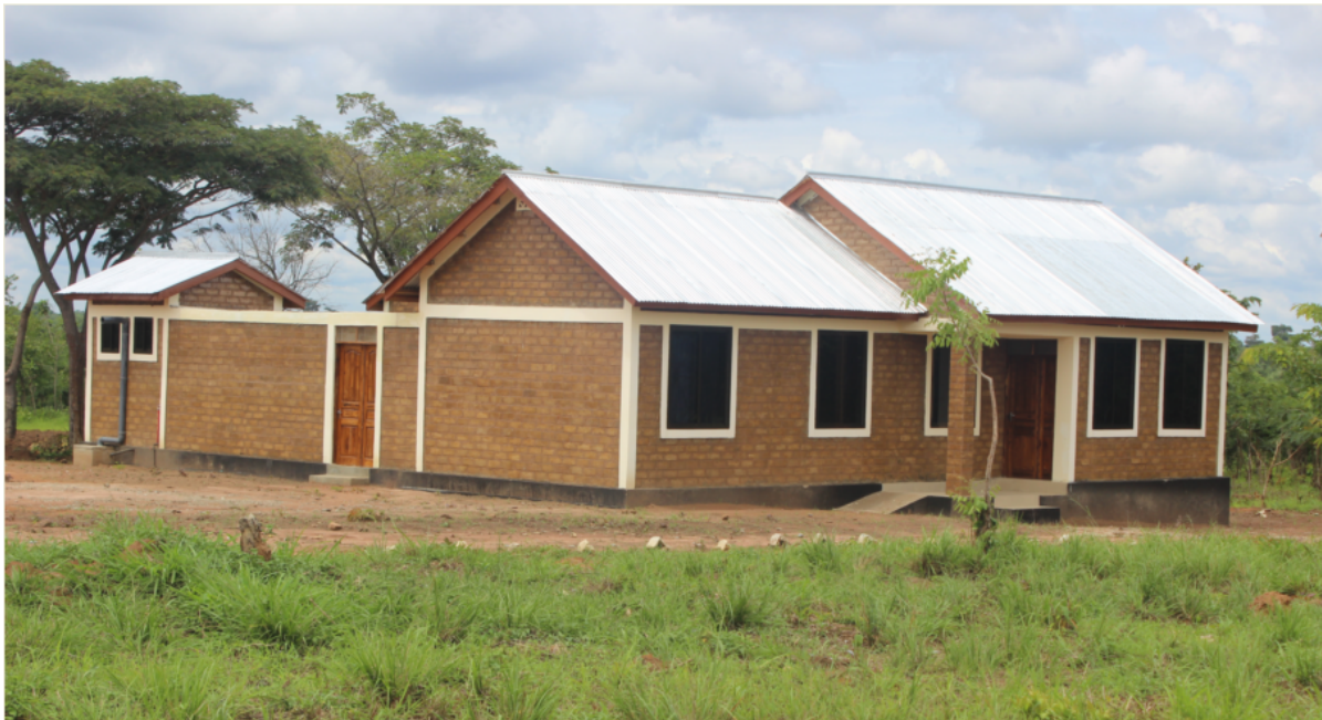
Figure 4 3-bedroom house in Tanzania, one of hundreds made of manually pressed, unmortared, stabilised-soil blocks
