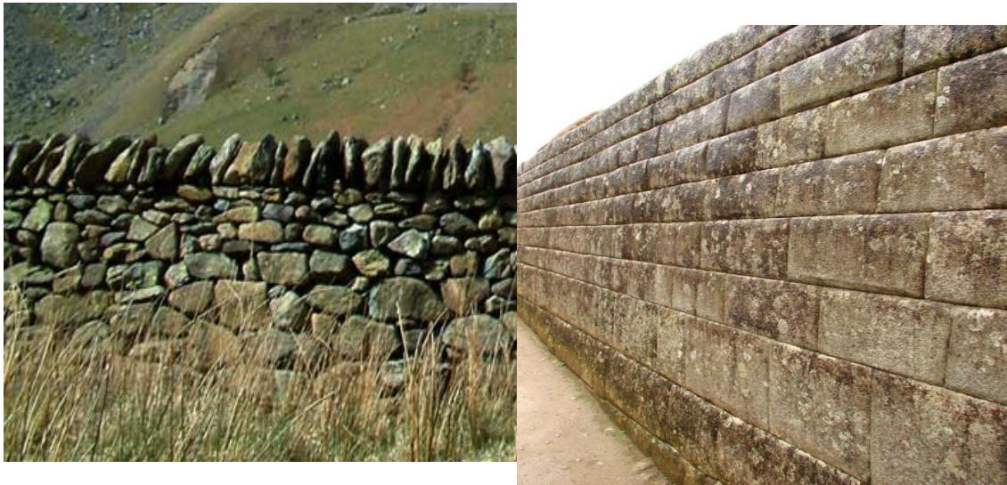
Figure 1 Drystone and ashlar walling.
