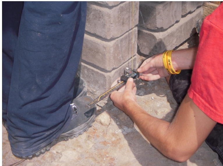
Figure 6 – Measuring out of plumb displacement using digital calipers
