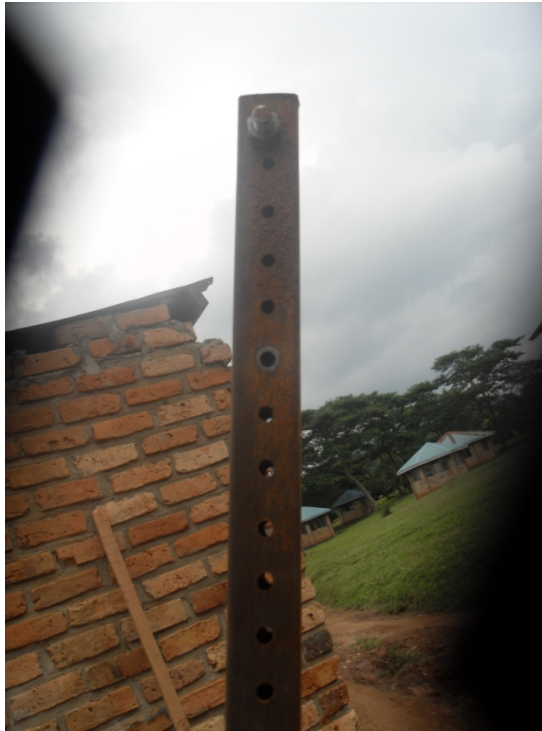
Figure 14 Holes in T-Bar at regular intervals
