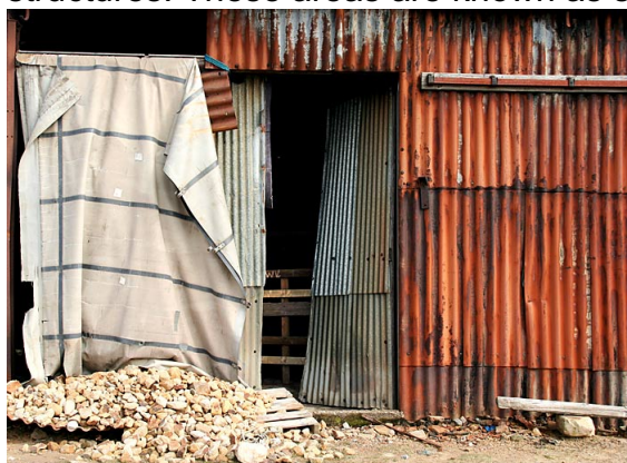
Figure 2 Corrugated iron shelter
