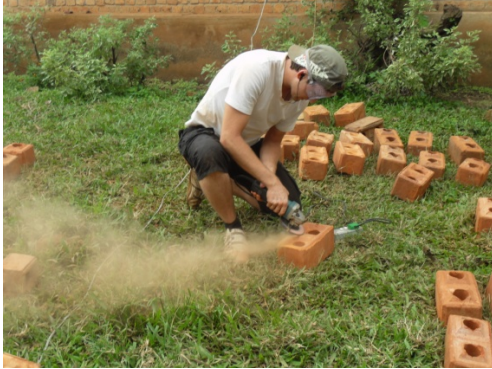
Figure 9 Using Anglegrinder on the bricks
