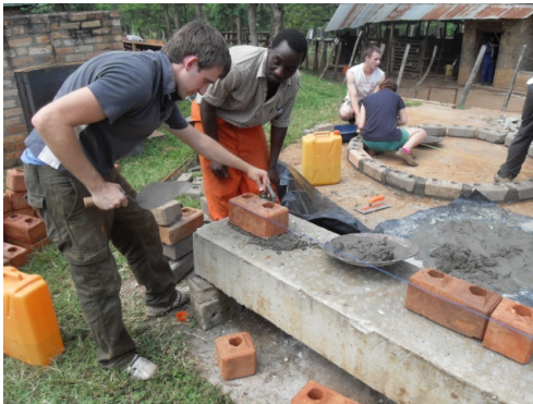
Figure 10 Placing the base bricks on the testing column
