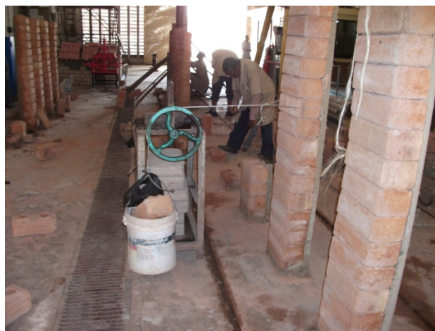
Figure 1: Bespoke Pulley System for Lateral Load Application
