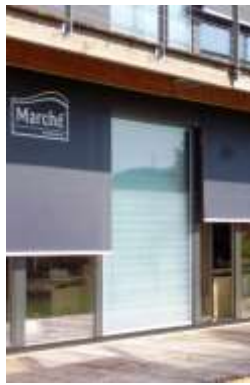
Exterior façade blinds combined with PCM (phase change) salts, Zurich. Source: author.
