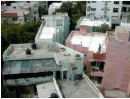
The World Bank “Cool Roofs” program. Painting concrete roofs white to reduce indoor temperatures – India. Source: www.cleanenergyministerial.org/GSEP
