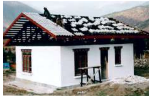
Microconcrete (MCR) roof tiles produced on site cheaper than CGI sheets; here also with a ventilated roof. Low cost houses, Bhutan, architect Chris Butters (source: author).
