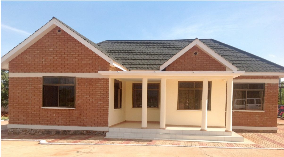
Tanzanian House made of Mortarless Interlocking Blocks of Stabilised Soil
