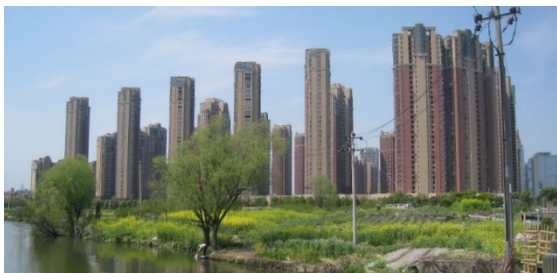
Typical residential high-rises, Ningbo, China
