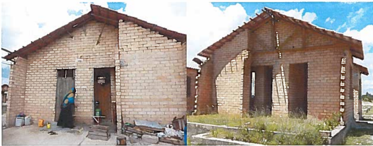
Figure.7. Completed and semi-completed NHBRA stabilised brick house (Author)
