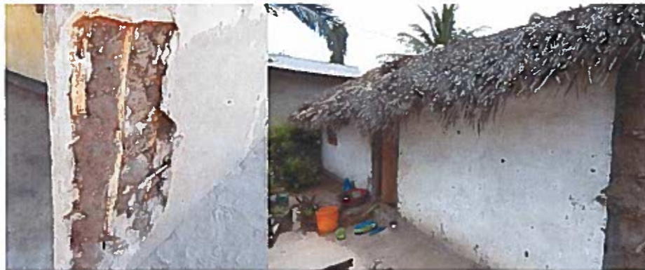
Figure.13. Plaster covered mud walls (Author)
