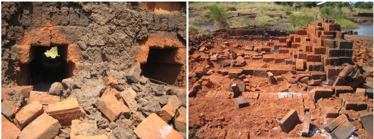
Figure 5: High material waste during production and handling (Tanzania).
