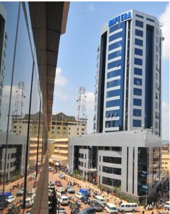
Mapeera house Kampala
