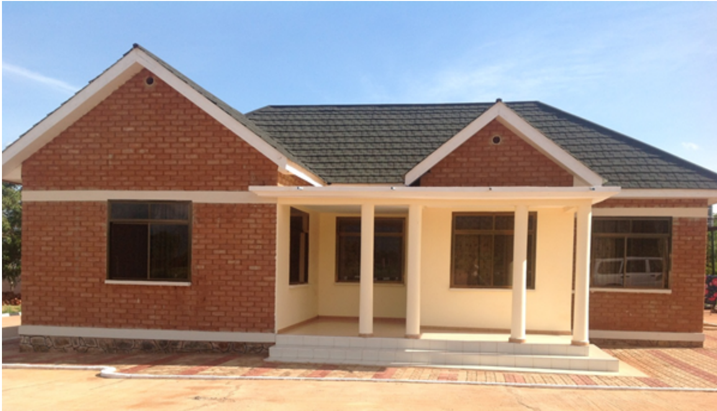
2 bedroom rural house in Tanzania – built of interlocking mortarless stabilised-soil blocks
