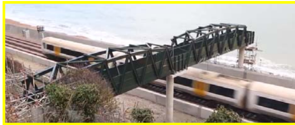
Dover sea wall footbridge, Dover, England (Pipex px)
