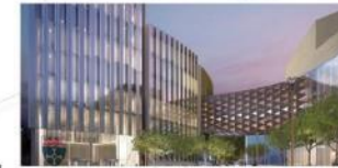
2) Learning & Teaching Centre Completion date: Autumn 2017
