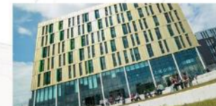
4) The Core Completed: November 2014
