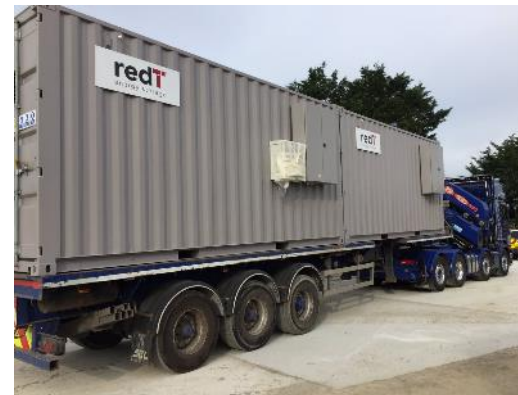
Commissioned redT 1.08MWh Redox Flow Machine at Olde House (Cornwall UK)
