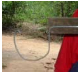
Bracket for mounting half round gutter onto eaves in Sri Lanka (Picture: B. Martinson)
