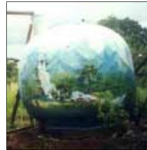
Ferrocement "pumpkin" tank in Sri Lanka (Photo T. Ariyananda)
