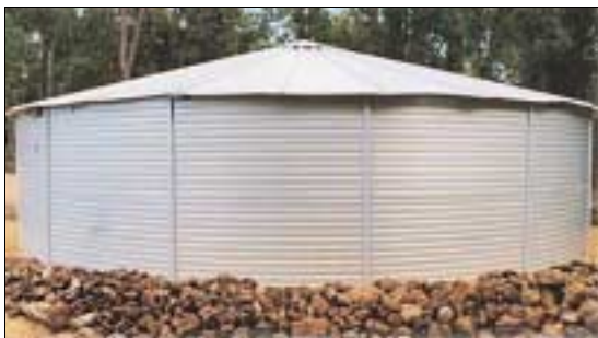
A large steel tank in rural Australia (Picture: Pioneer Tanks Pty. Ltd.)
