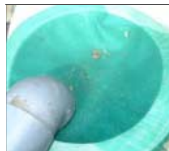
Course leaf filter at tank entrance in Sri Lanka (Picture: B. Martinson)
