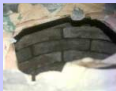
Made up mould (Picture: R. Ariyabandu)
