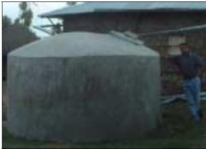
Household ferrocement tank in Ethiopia (Picture: S. Akhter)
