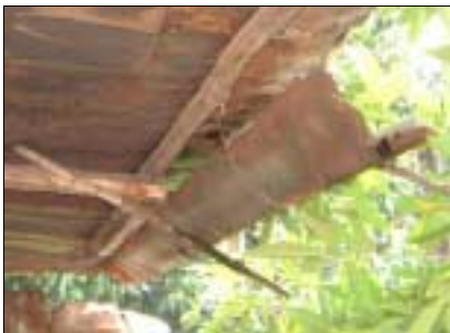
Ad-hoc mounting of vee shaped gutter using wires and roundwood in Ethiopia (Picture: S. Akhter)
