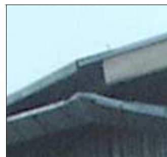
Vee shaped gutters with splash guard in Ethiopia
