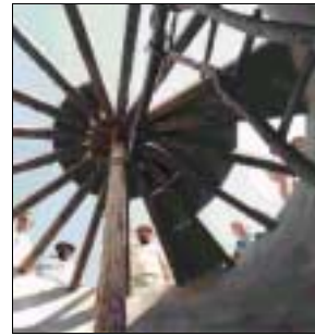
Precast plates being placed on a ferrocement tank in Brazil (Picture: Johann Gnadlinger)
