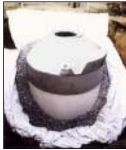
A precast concrete tank being buried in urban Germany (Picture: Mall GmbH)
