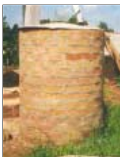
Tank made from stabilised soil blocks in urban Uganda (Picture: T. Thomas)
