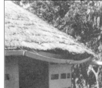
Round thatched roof in Kenya Note the bent guttering (Picture Lee and Visscher)
