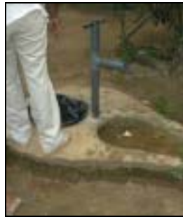
Tube tank made without overflow in Sri Lanka
