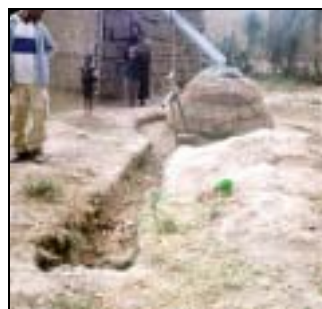
Good drainage practice on thatch tank in Ethiopia
