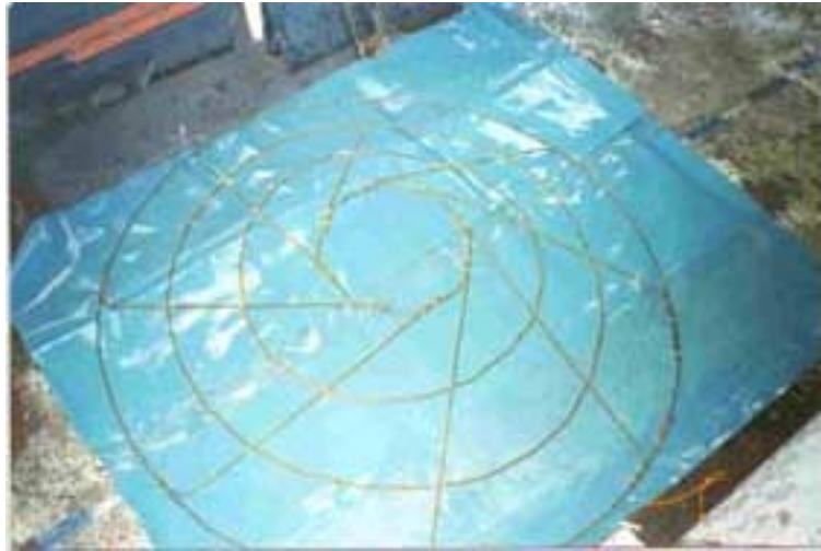
Figure 7. The frame with hoops in place.
