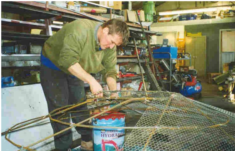
Figure 10. Applying the chicken mesh.
