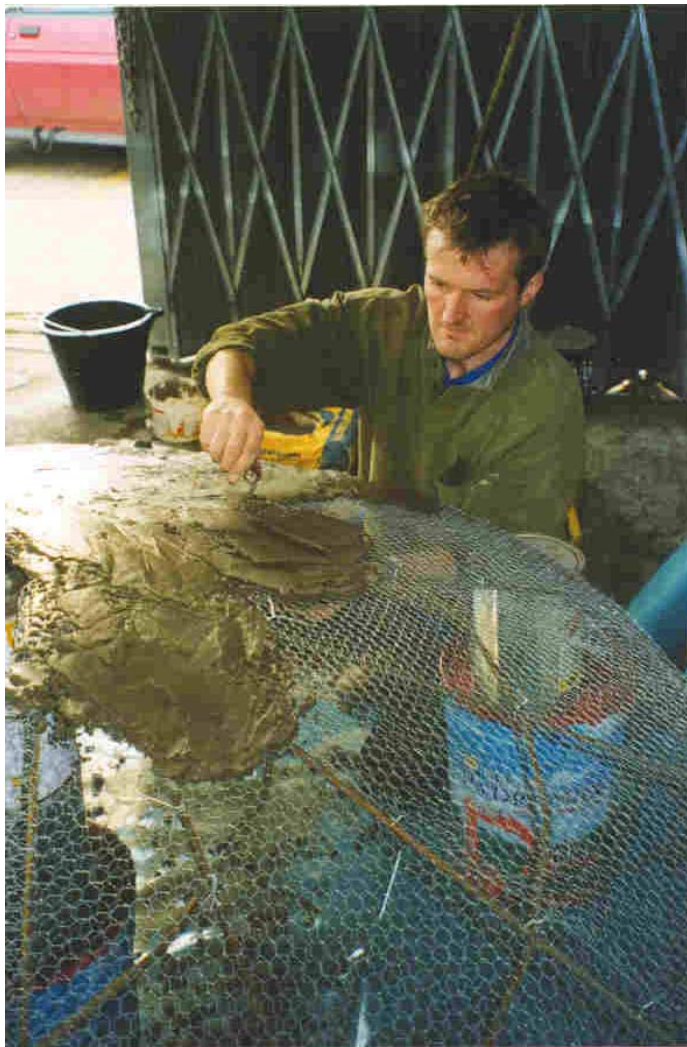
Figure 12. Applying render to the chicken mesh.
