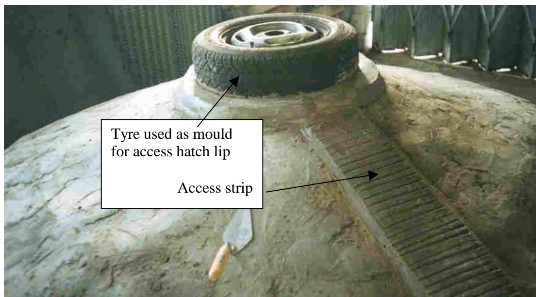
Figure 13. Showing finished access strip and old tyre used as former for access hatch lip.
