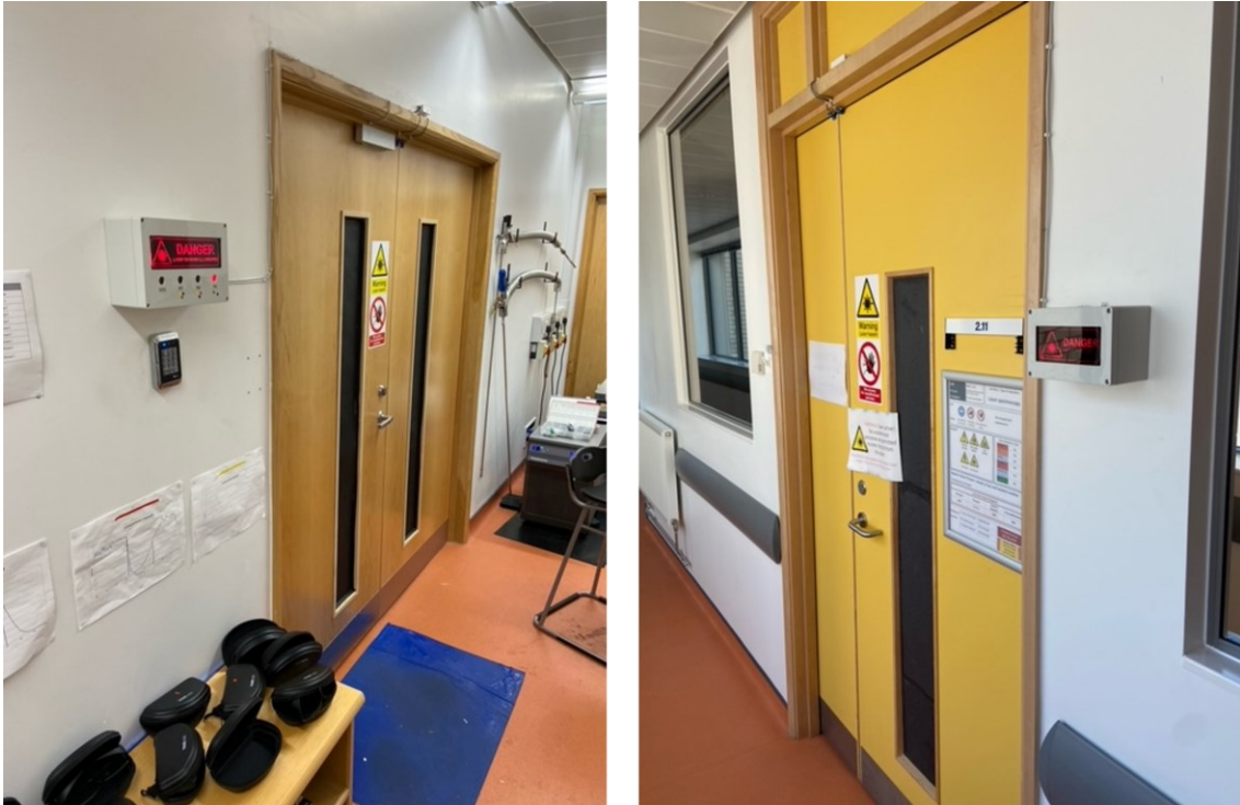
Figure 1: Pictures of both entrances to the facility. Left shows the main entrance inside the annex with the magnetically interlocked door, warning light and appropriate signage. Right, shows the rear door to the lab (which is kept locked) with warning light and appropriate signage.
