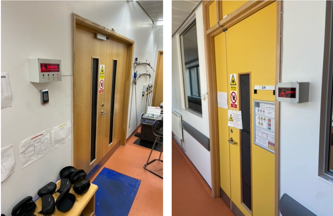
Figure 1: Pictures of both entrances to the facility. Left shows the main entrance inside the annex with the magnetically interlocked door, warning light and appropriate signage. Right, shows the rear door to the lab (which is kept locked) with warning light and appropriate signage.
