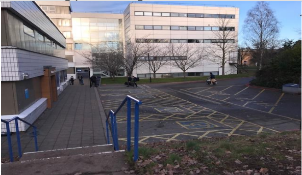
Unfenced drop onto the car park.
