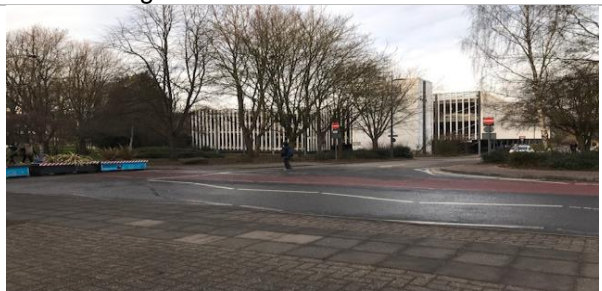
Multi Storey Carpark located across the road
