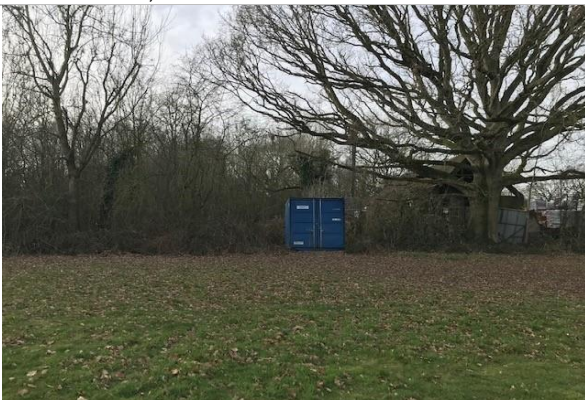
Container unit integrated into the boundary.
