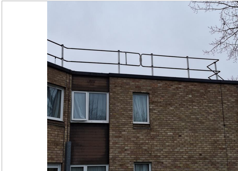
Roof access gate
