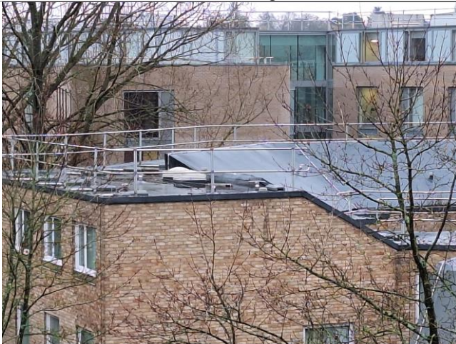
Roof incline and sky lights
