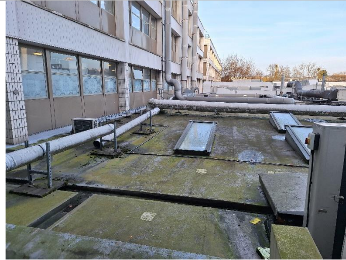
Roof layout including sky lights and pipework
