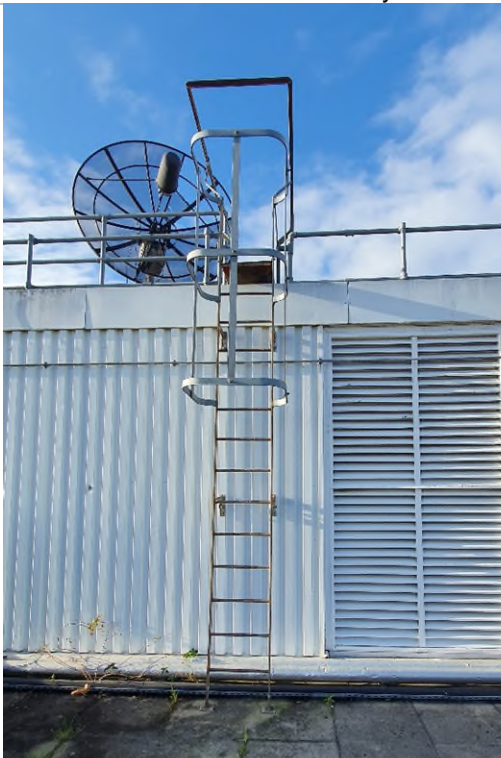
Access ladder to upper roof and departmental antenna
