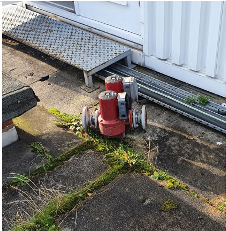
Discarded pump set
