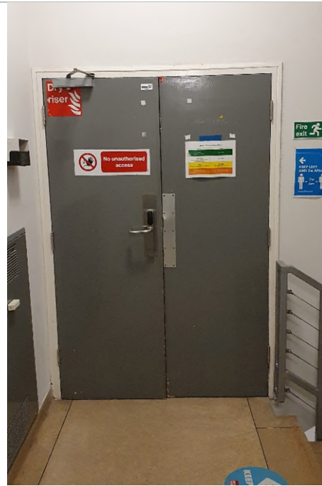
Plant room door on 5 th floor
