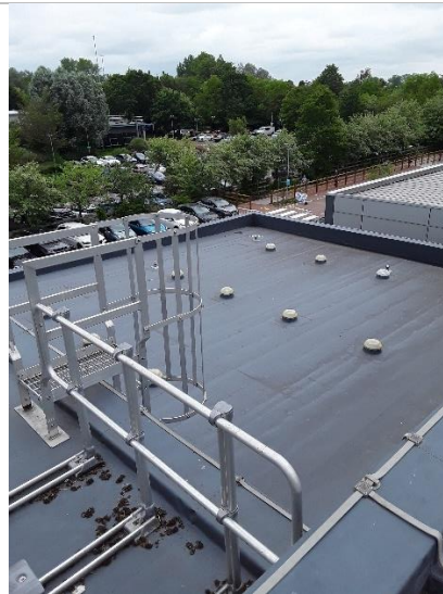
Upper-level roof view
