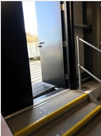
Salto access door leading to the roof external area on the 2 nd floor.
