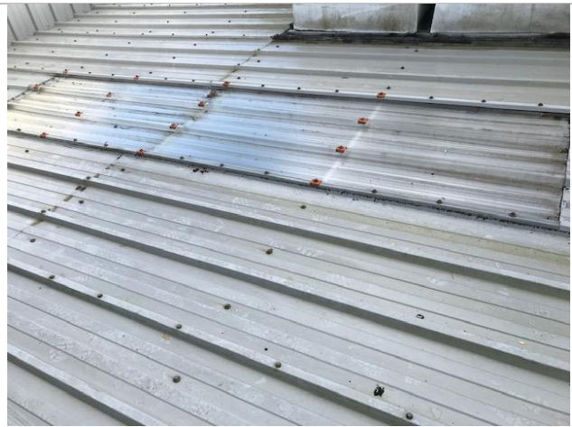
Skylight on the roof
