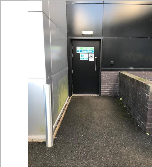
Black door with Salto access leading to the stairs to access the roof.
