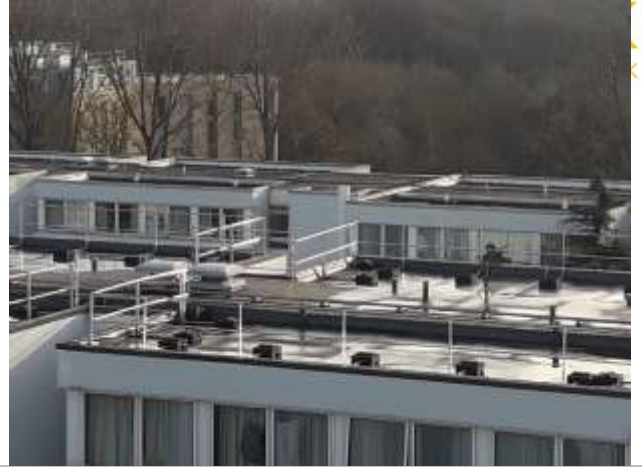
Roof Staging area
