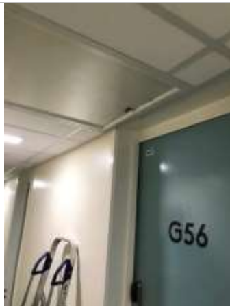
Ceiling Hatch Location
