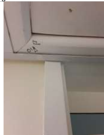
Ceiling Hatch Location
