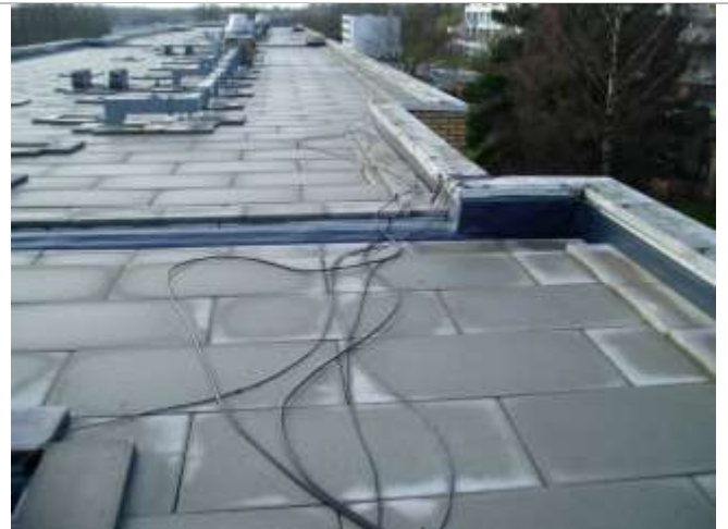
External roof area
