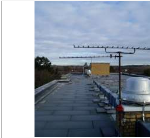
External roof area
