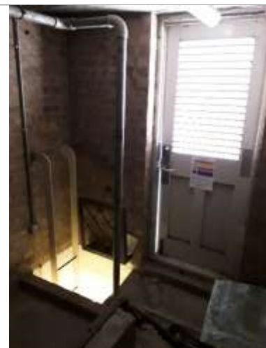
Galvanised ladder leading to door to access flat roof.
