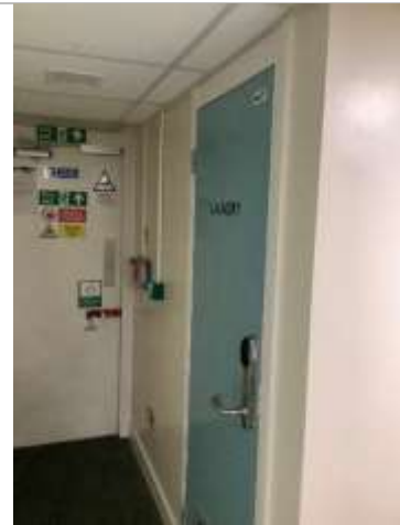
Laundry room door leading to roof hatch
