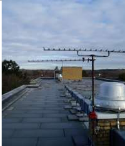
External roof staging area
