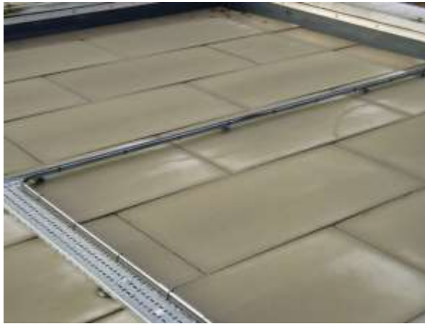
External roof area
