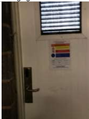
Door leading to roof with Salto access
