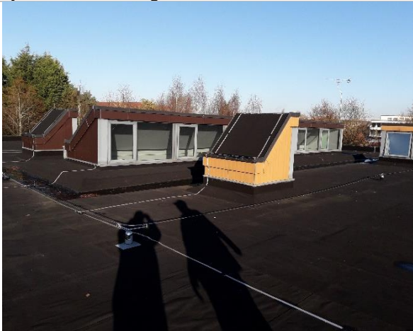
Eyebolts at the edge of the roof to fix ladder
