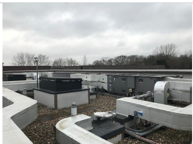
Cryfield 15 external roof area
