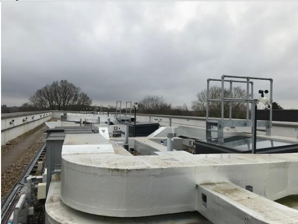
Cryfield 11 External roof.
