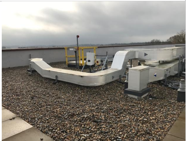
Cryfield 10 roof staging area
