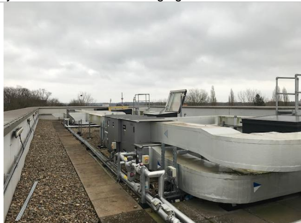
Cryfield 12 external roof staging area.
