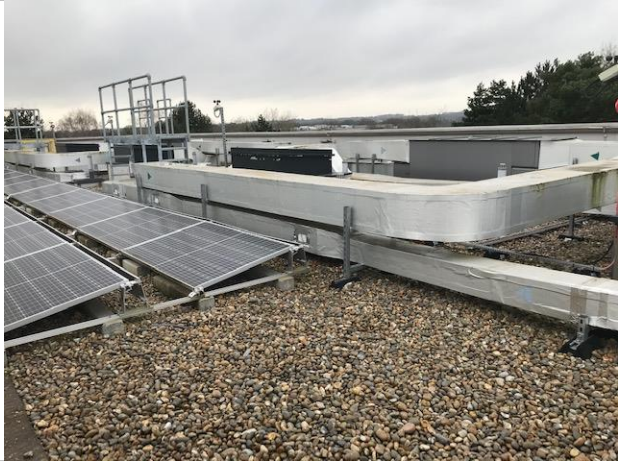
Cryfield 14 external roof area
