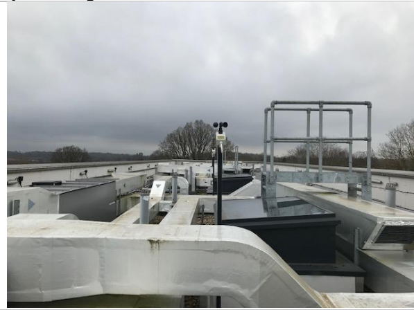
Cryfield 11 External roof
