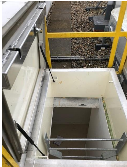
Cryfield 15 roof hatch access
