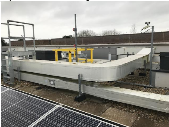
Cryfield 12 external roof staging area.
