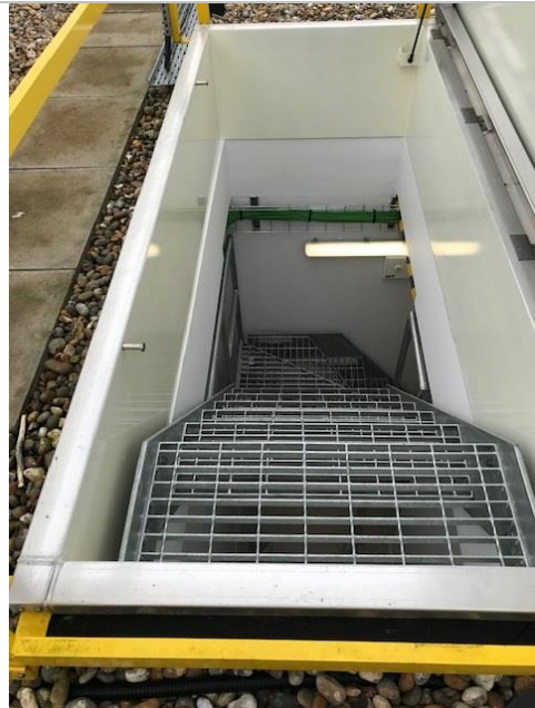
Cryfield 11 galvanised staircase to roof
