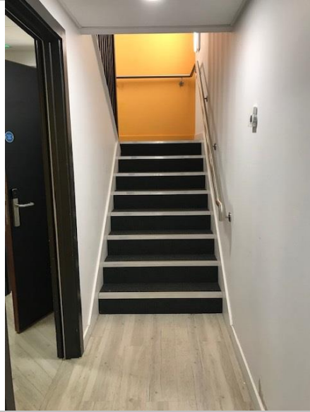
Cryfield 11G stairs to access roof
