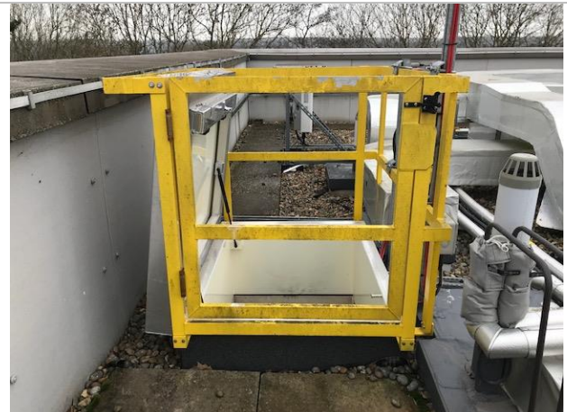
Cryfield 13 roof hatch access
