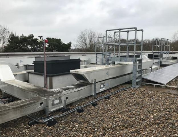
Cryfield 14 external roof area
