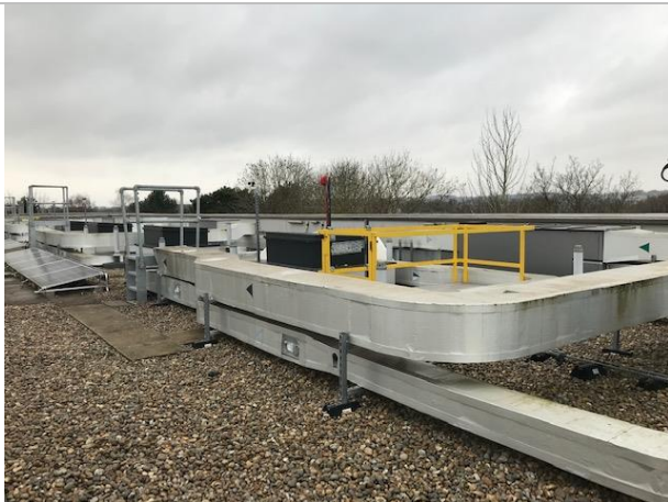
Cryfield 13 external roof.
