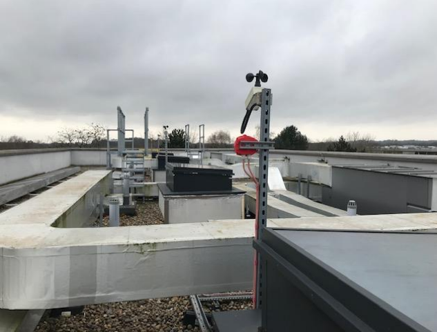
Cryfield 14 external roof area
