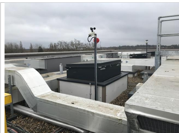
Cryfield 15 external roof area
