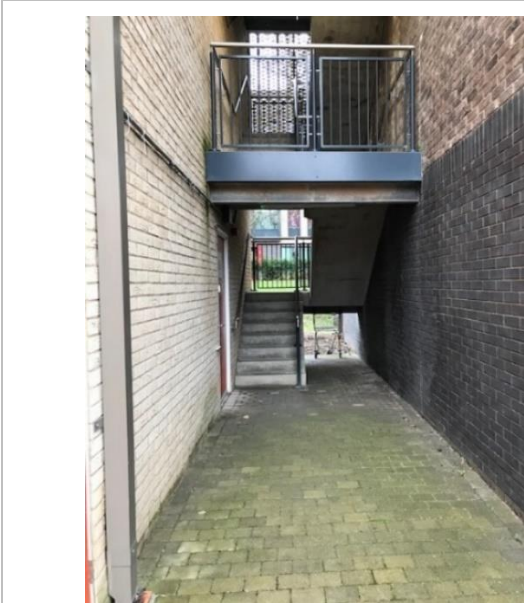
Cryfield 12 Ground floor external staircase access.
