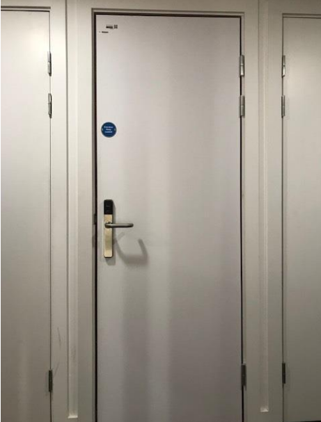
Cryfield 14 door to access roof.
