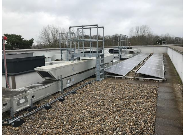
Cryfield 14 external roof area
