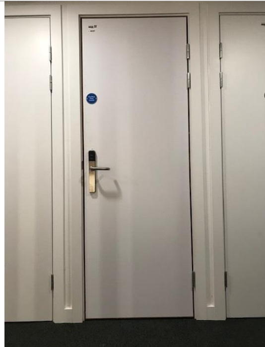
Cryfield 15 door to access roof.
