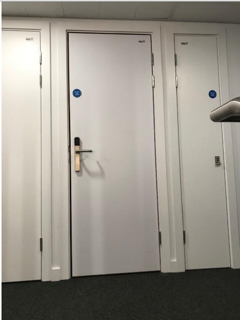
Cryfield 11 Door to access roof.
