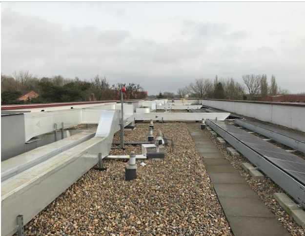
Cryfield 10 roof staging area
