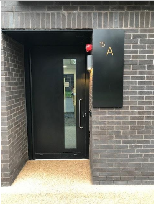
Cryfield 15, Apartment 15A to access the roof.
