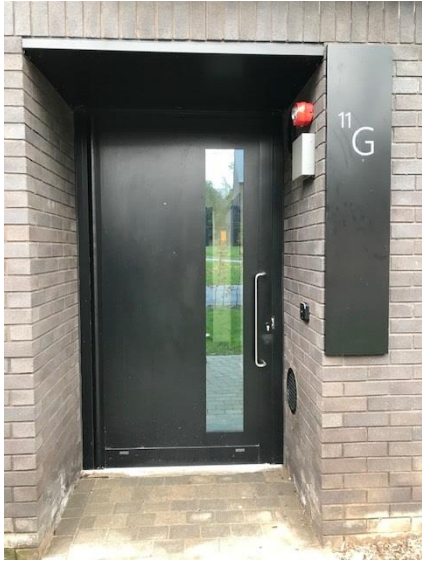
Cryfield 11, Apartment 11G entrance to access roof
