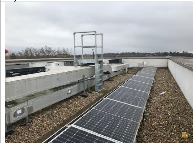
Cryfield 15 external roof staging area
