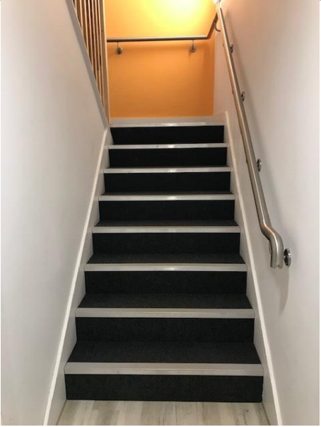
Cryfield 14, stairs leading to third floor to access roof.
