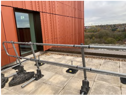
There is a gap of around 2 metres between the edge protection and the edge of the building.
