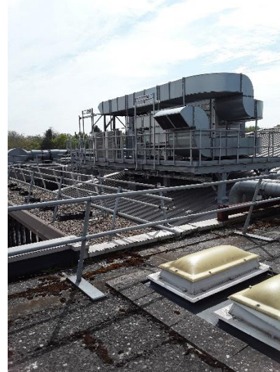
Edge protection, sky lights and plant
