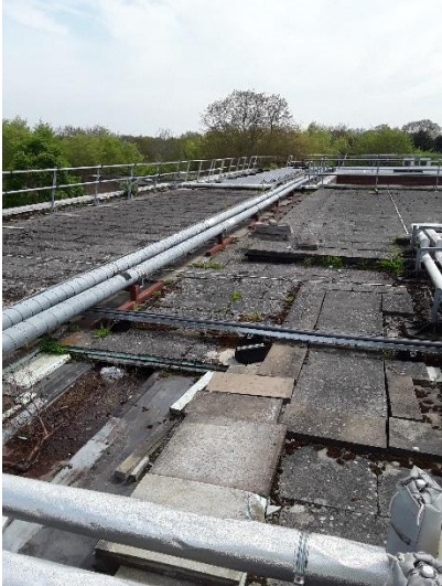
Area where gantry is required to access roof
